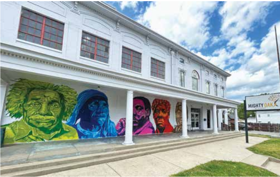
Mighty Oak Academy, 26th Street in the old Mackin building
