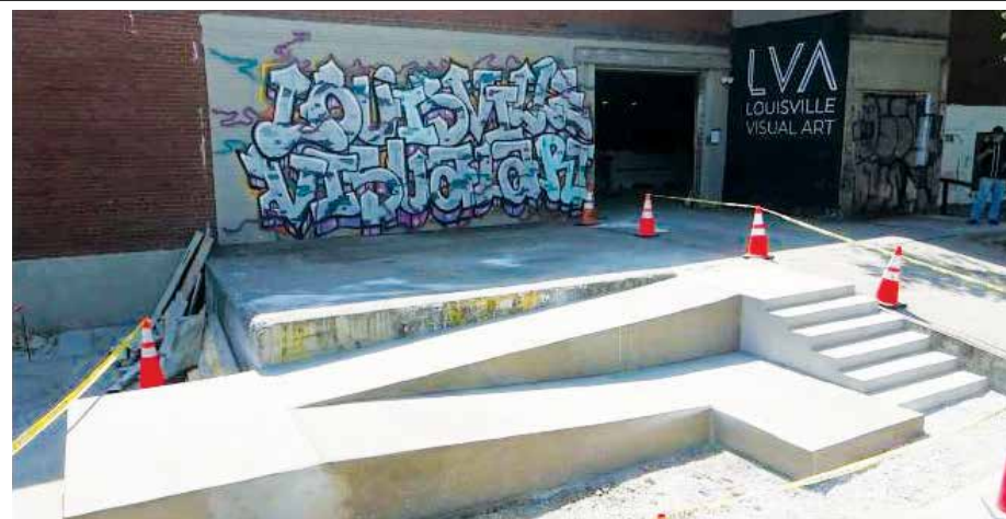
The newly-poured exterior steps and ramp at 1538 Lytle Street, LVA's headquarters.
