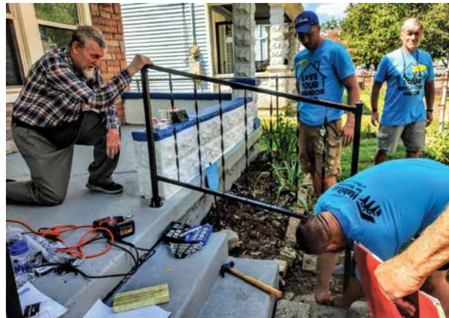
Homeowner get new railing installed on porch steps.
